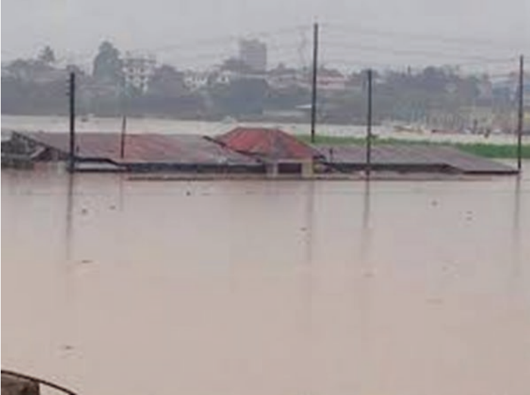
Fig. 9.7 Electricity infrastructures covered by water
