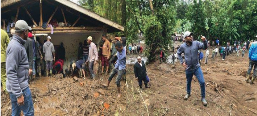
Fig. 9.10 Reconstruction of houses after floods
