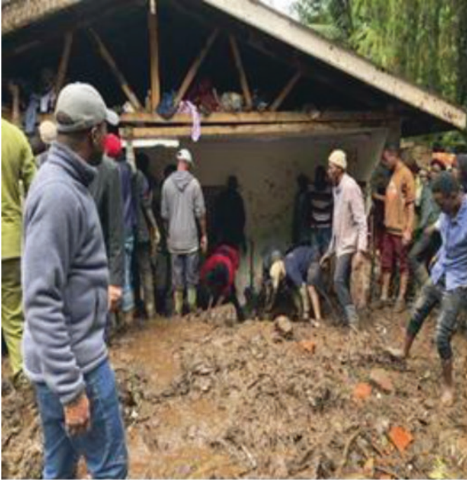
Fig. 9.3 Reconstruction of houses after floods
